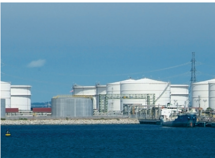
TANK STORAGE & TERMINALS
